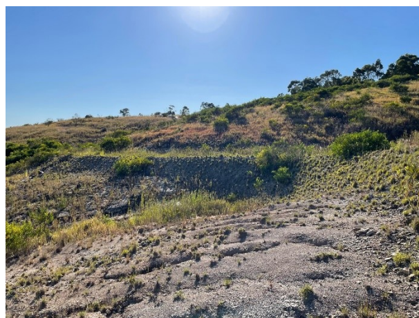
Access track bisecting site with a batter up to 35°.
