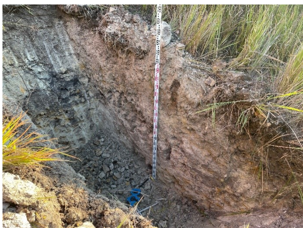
TP11 was excavated on the upper slope of the northern face of the spur and encountered colluvial soil overlying very low strength tuffaceous material overlying medium strength sandstone.
