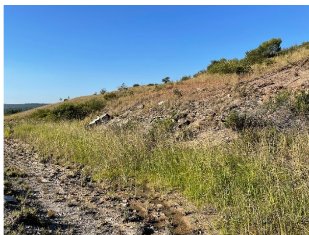
Access track constructed through the site with water pooling.
